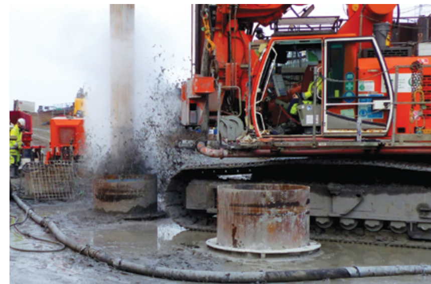
Piling work for the Target building
