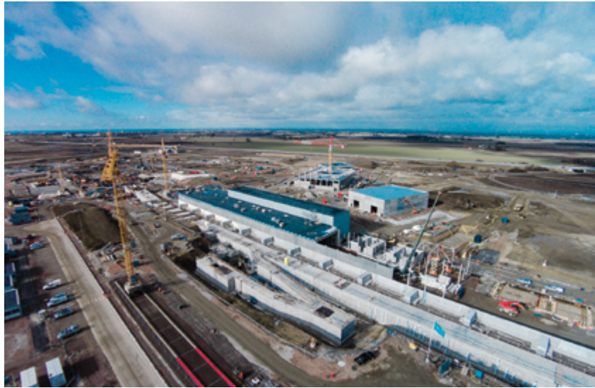
The Accelerator tunnel taking shape
