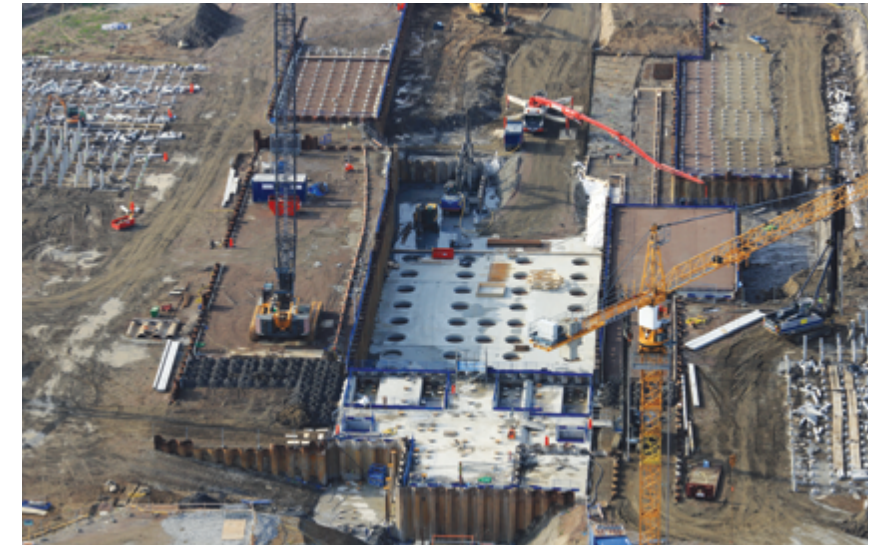
Piling works for the Target
