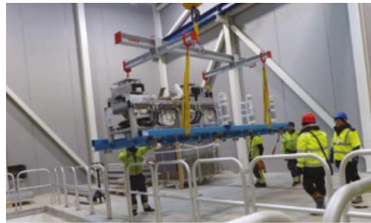
*The ESS high-intensity proton source and LEBT line at INFN-Catania, where it was designed and commissioned*
